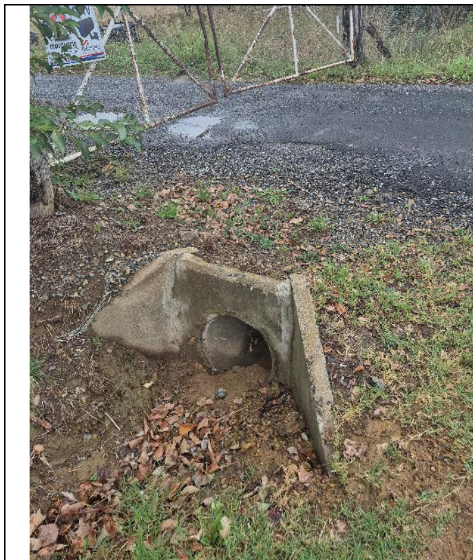
Figure 31: site inspection photo – existing vehicle access crossing
