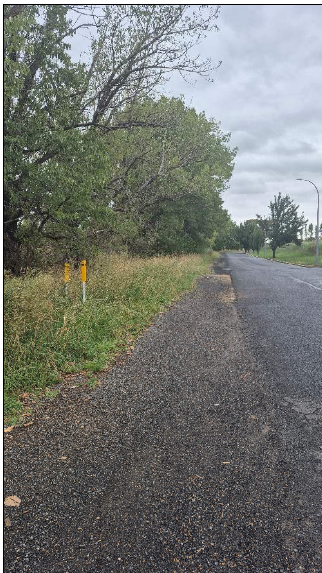
Figure 30: site inspection photo: - extent of pavement on Perc Griffith Way
